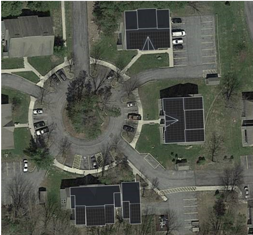
Figure 2. Aerial photo of buildings 1, 2, and 3 at the Christopher Court complex with the solar PV panels laid out for spacing and size
